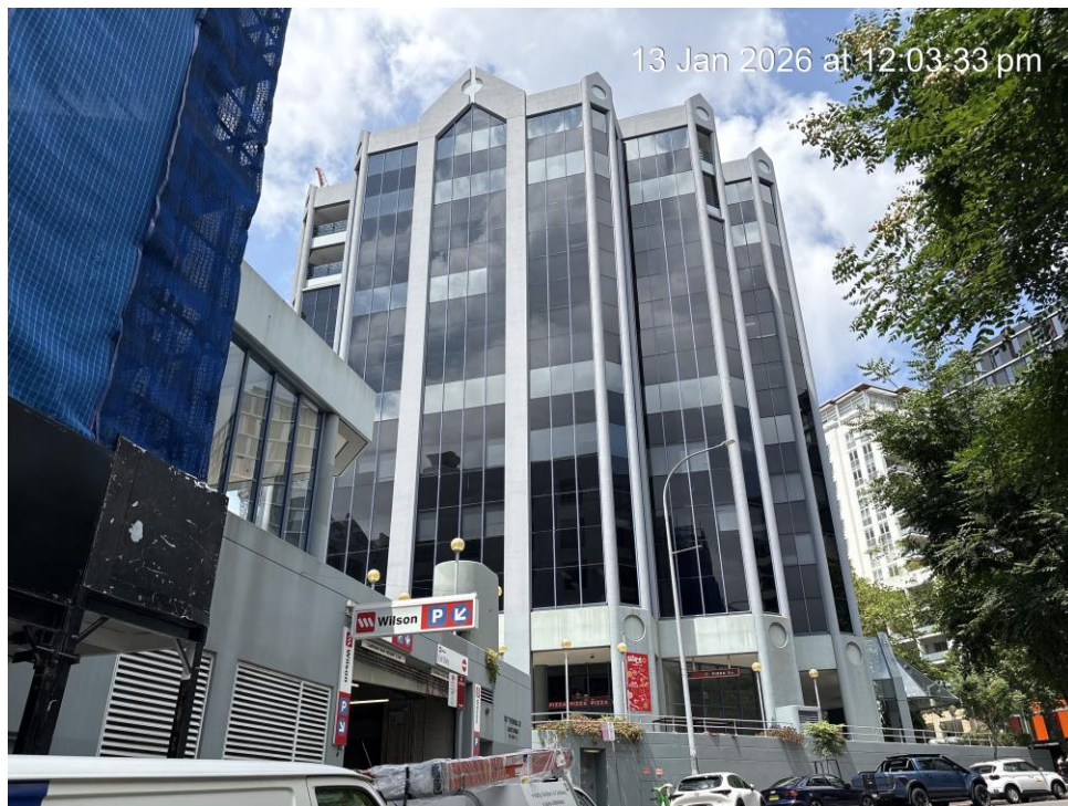
Figure 1: 187-189 Thomas Street, Haymarket viewed from the north-west
